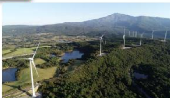
Nikaho No.2 Windfarm
