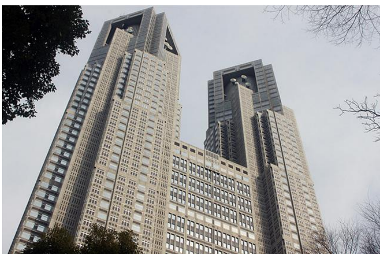
TMG No.1 Building
