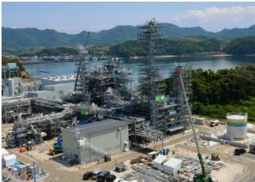
CO 2 Capture Facilities of Osaki CoolGen under Construction
