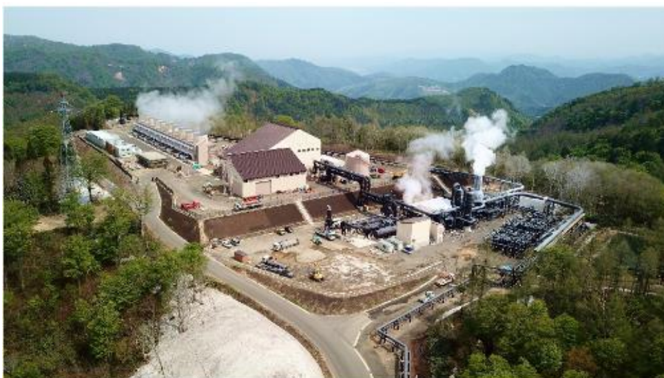
Whole view of Wasabizawa Geothermal Power Plant
