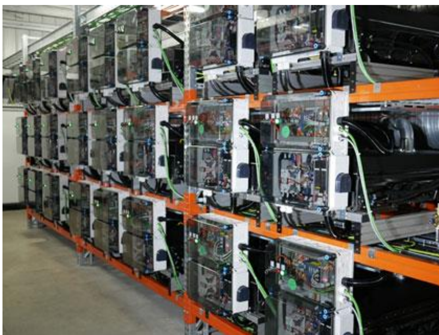
The Mobility House manages energy storage systems consisting of EV battery packs https://www.mitsui.com/jp/en/release/2017/1224845_10832.html
