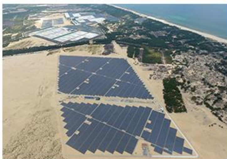
Completed Mega Solar Power Plant
