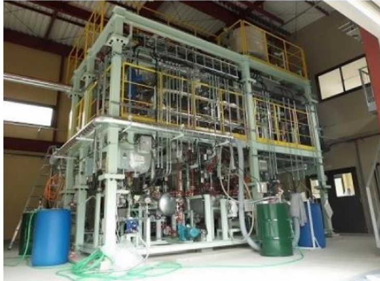
Research facilities on bioplastic materials
